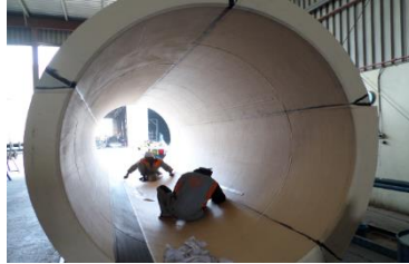
application of rubber lining layers
